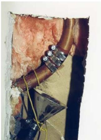
**Fig 1** – Rubber hose clamped on a leaking cold bend in copper pipe (tubing). The leak was so pervasive that a funnel was installed to remove the water drip. This is not long-term management of copper tube corrosion.
