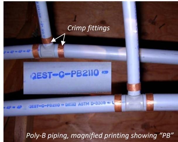
Common failures with Poly-B piping center around the polybutylene material's sensitivity to both temperature and chlorine, both common in hot water systems. Over time the piping is chemically degraded (weakened) and fails under system pressure. This degradation occurs on the inside wall of the pipe, meaning piping can be dangerously degraded, but look perfectly normal on the outside.
