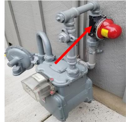
Figure 1. Typical installation of seismic shutoff valves.
