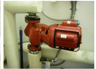
CIRCULATING/RECIRC. PUMPS
