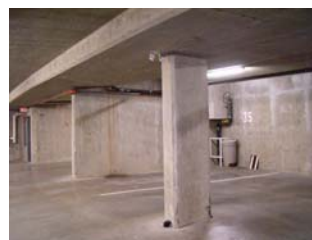
CONCRETE COLUMNS IN PARKADE
